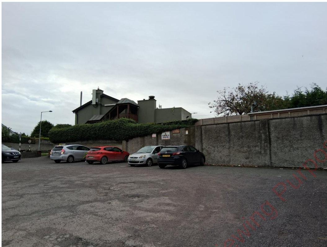
Figure 5 – Shows the existing 2.1m wall between the car parking area and beer garden no. 2.
