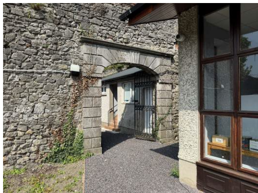
Protected Structure – east elevation
