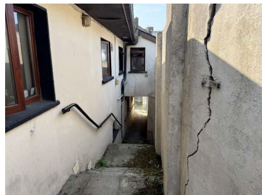
Pedestrian stepped link to West Street
