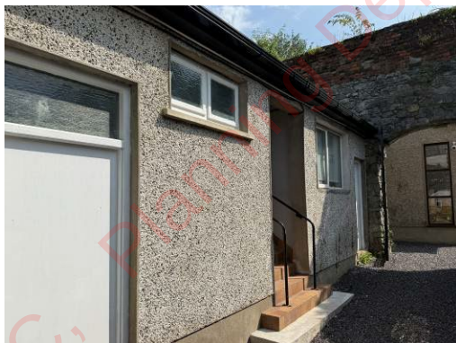
Toilet Block – Arch in background
