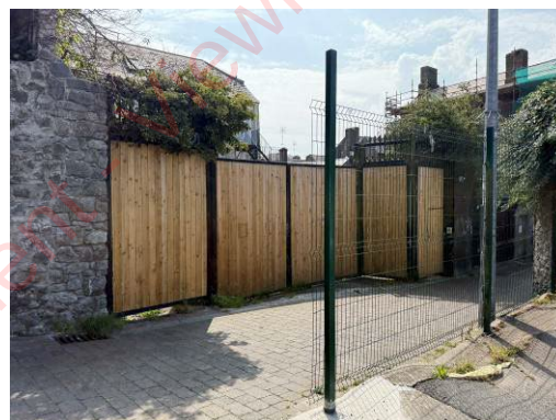
Site Entrance / Gates from Scholes Lane
