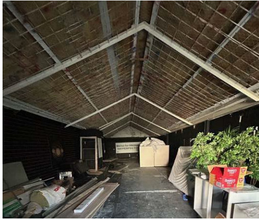
Retail Unit – Interior View
